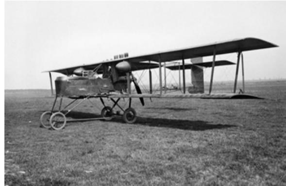
Figure 4 The unmanned aircraft Voisin BN3<sup>9</sup>
