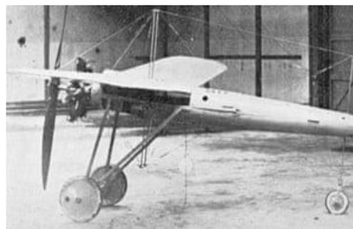
Figure 1 Ruston Proctor Aerial Target<sup>3</sup>
